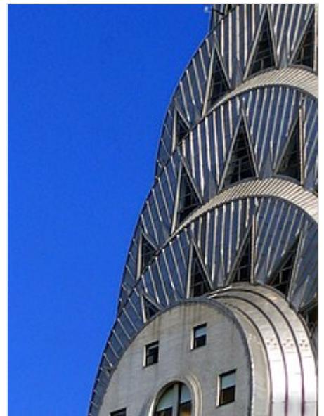
The pinnacle of New York's Chrysler Building , the world's tallest steel-supported brick building, is clad with stainless steel.
